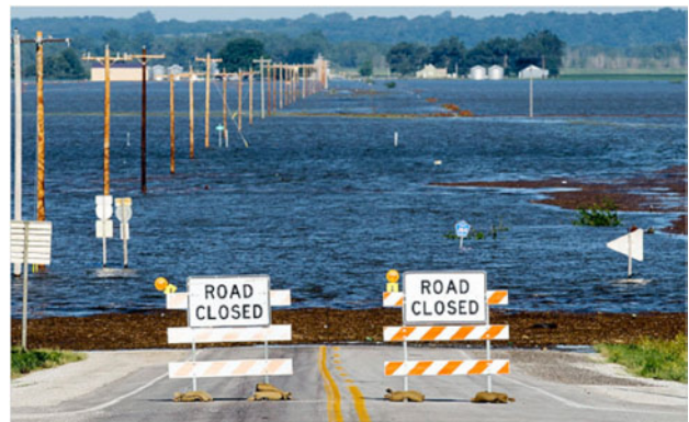
Damage caused by the 2011 Mississippi flood
